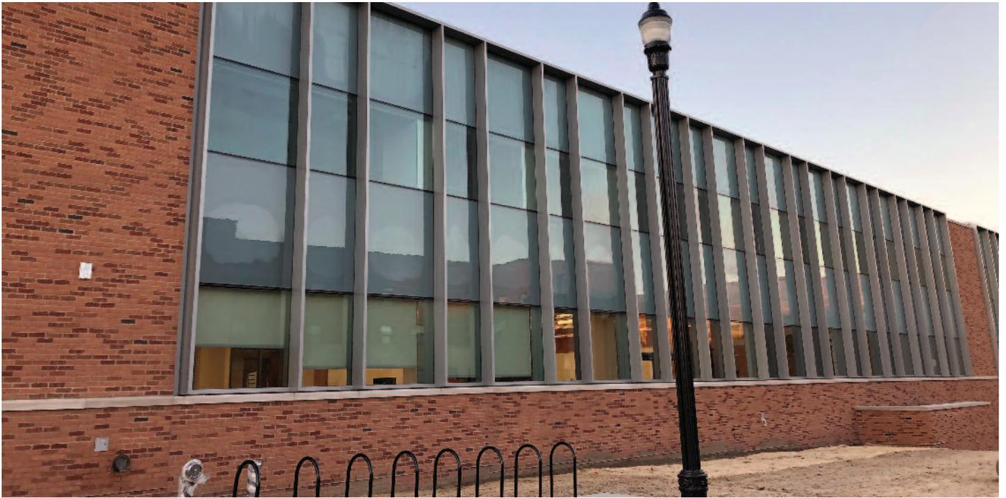
Exterior building materials – brick and aluminum/glass curtain wall – were selected to harmonize with the other buildings of the science complex, and were detailed for durability and energy efficiency.
